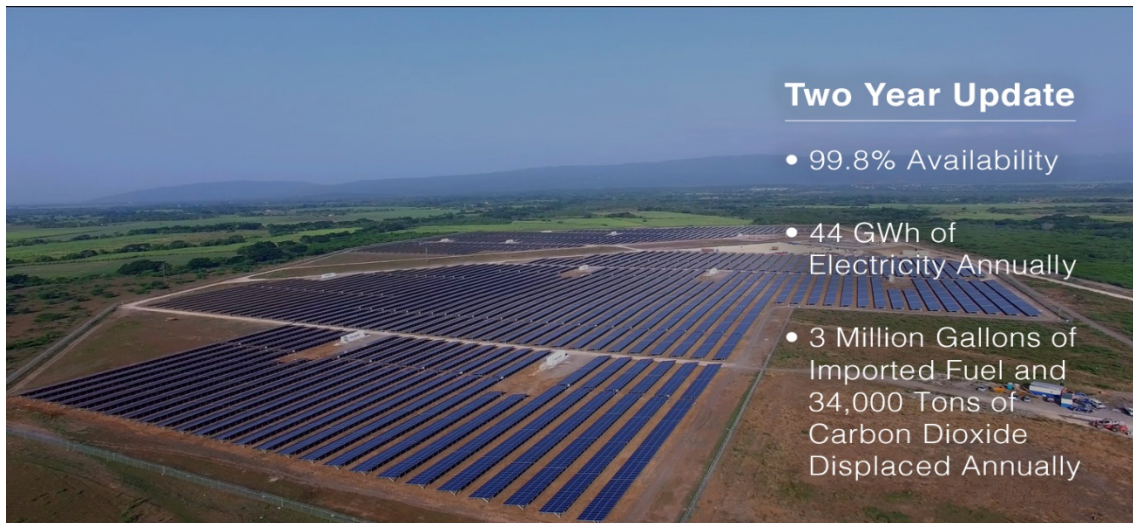
Aerial view of 160-acre Content Solar PV power plant in Clarendon, Jamaica
